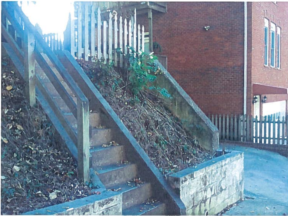
Fig. 2 - Existing concrete steps from Greenwood Avenue.
