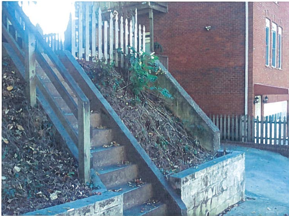
Fig. 2 - Existing concrete steps from Greenwood Avenue.
