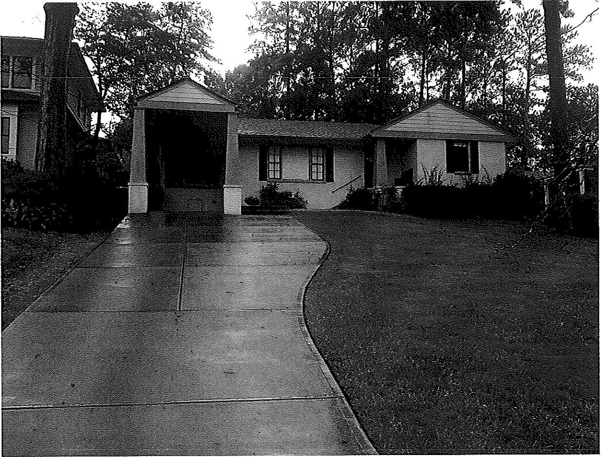
Carport @ 1215 Spring Valley Lane. 2 houses down from 1227.
