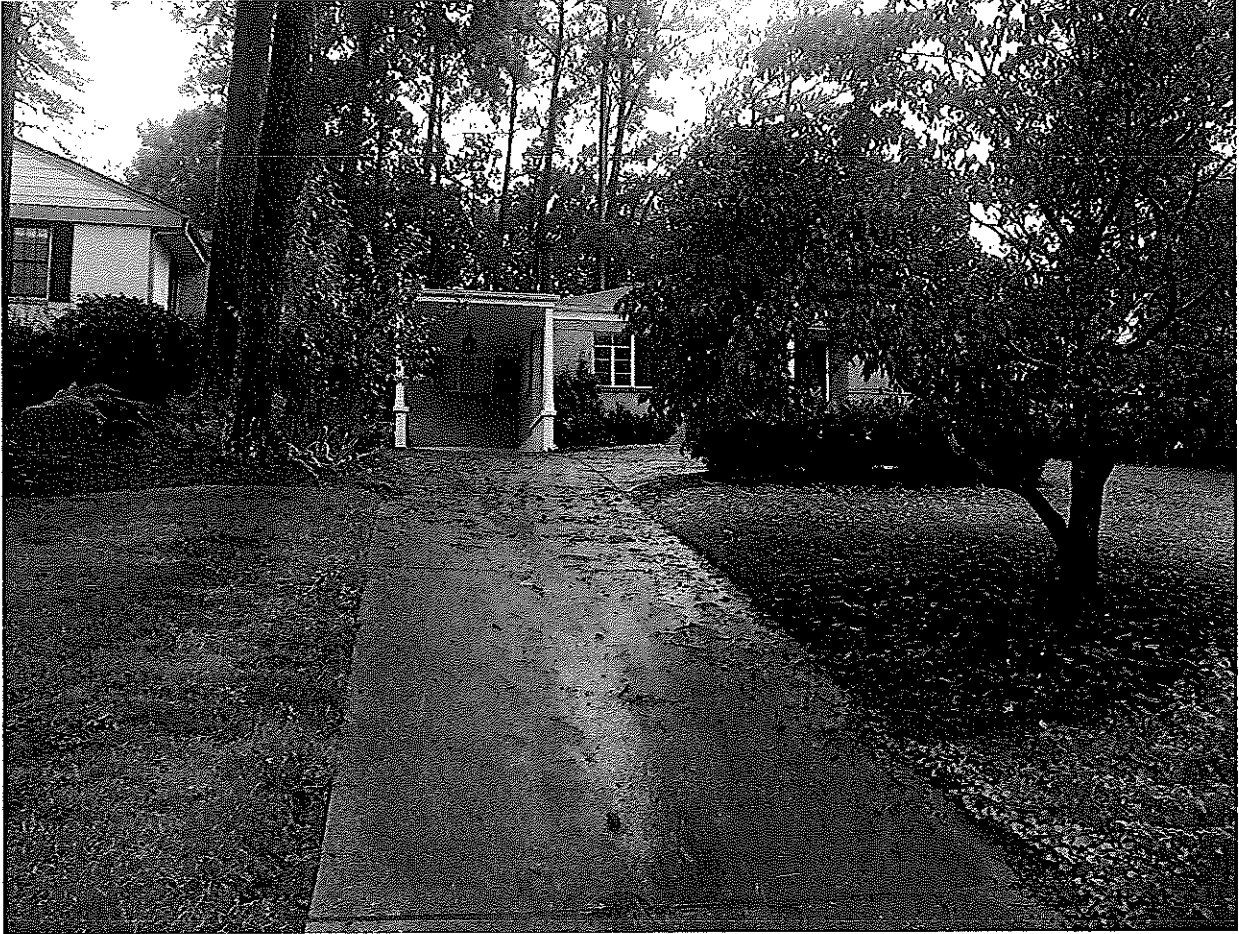
Carport @ 1209 Spring Valley Lane. 3 houses down from 1227.
