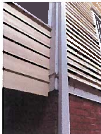
Detail at screened porch and existing House
